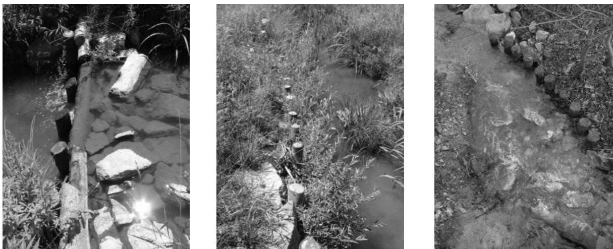
*Figure 3: Revitalization measures in a small stream: weir (left), willow knit (middle) and flow deflector (right)*
